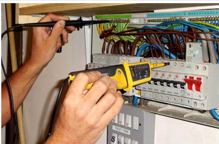
Completing electrical installation testing as per BS7671
