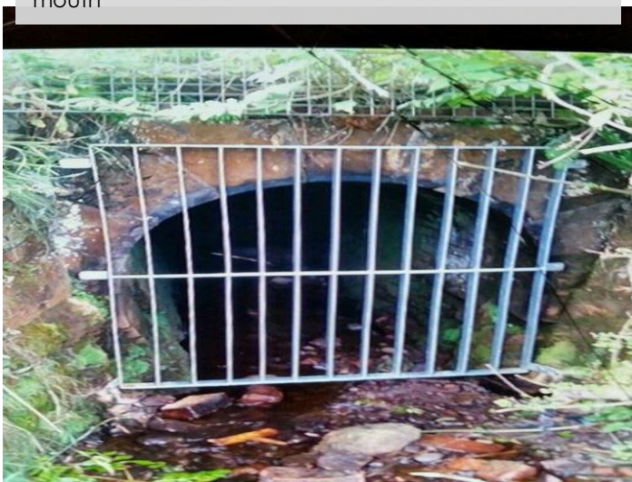
Completed galvanized steel grating fixed to culvert mouth
