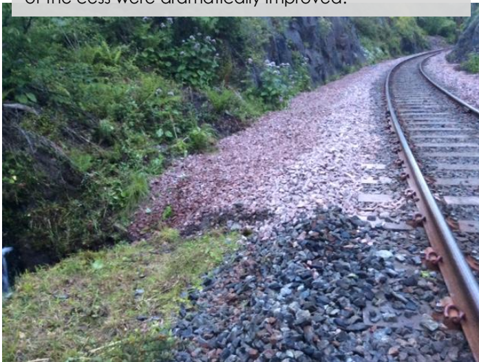
Upon completion of the works, the ground conditions of the cess were dramatically improved.
