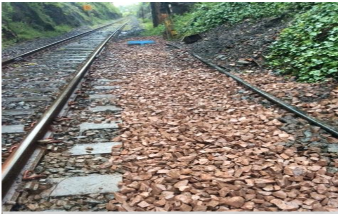
Upon completion of the works, the ground conditions of the cess were dramatically improved.
