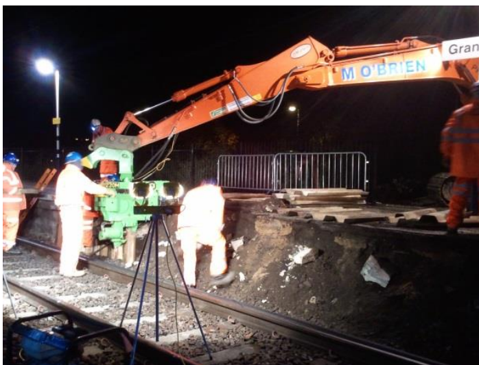
Traditional Harp unit platform construction
