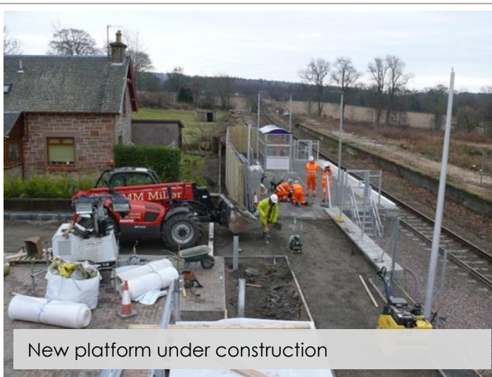
Ballast retention using sheet piles
