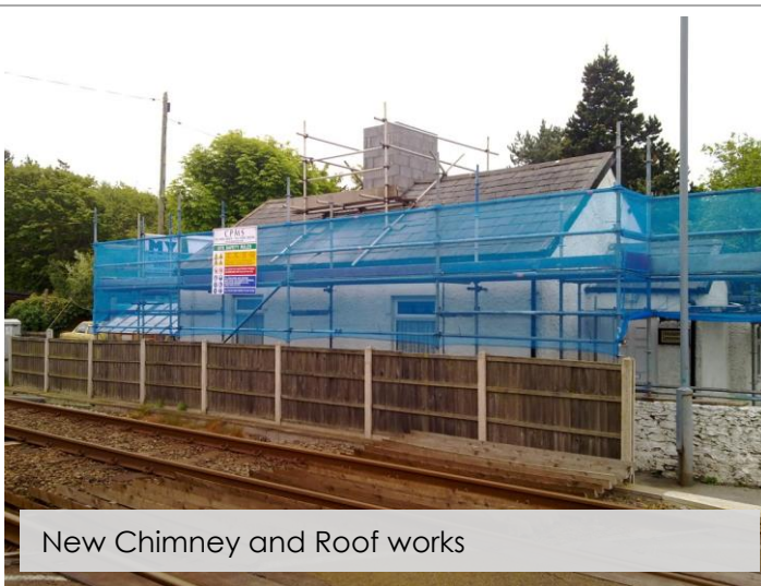
Down taking of Train Maintenance Shed for reuse
