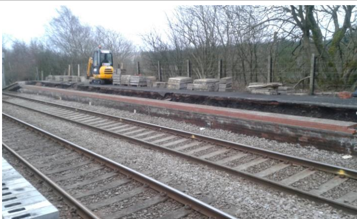
Platform wall removed and rebuilding commenced
