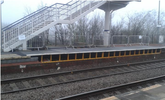
Temporary platform construction
