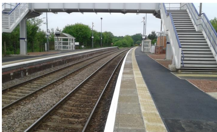
Rebuilding of platforms complete
