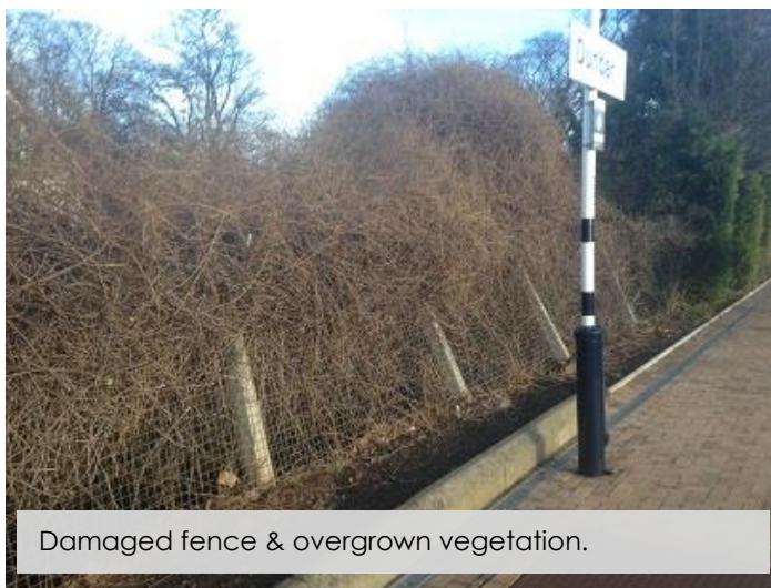
Damaged fence & overgrown vegetation.
