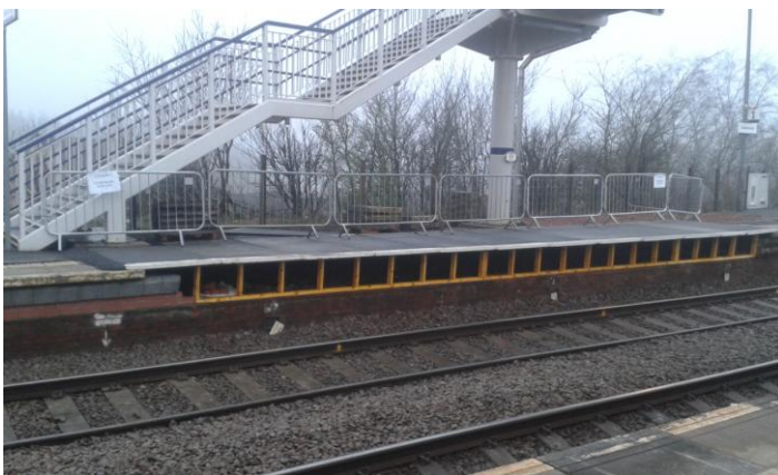
Temporary platform construction
