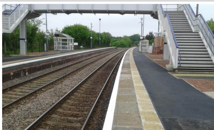
Rebuilding of platforms complete
