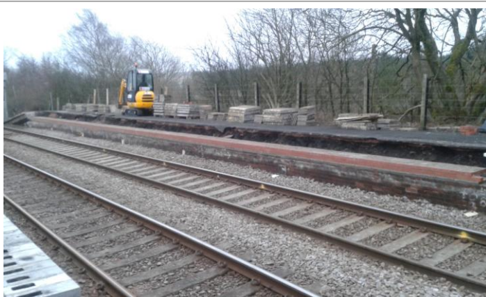
Platform wall removed and rebuilding commenced
